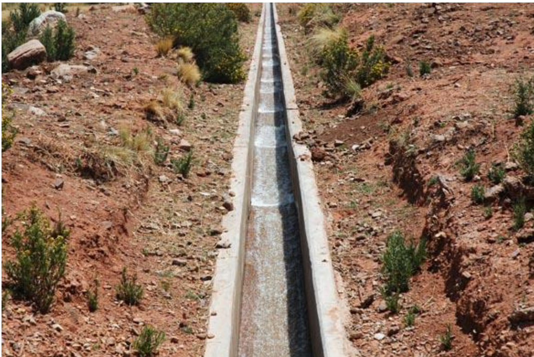
Figure 1. Roll waves in irrigation canal, Cabana-Mañazo project, Puno, Peru.
